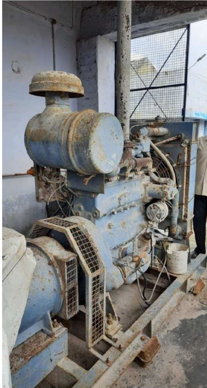
Fig.7.5 Picture of an engine generator or genset running on diesel.
